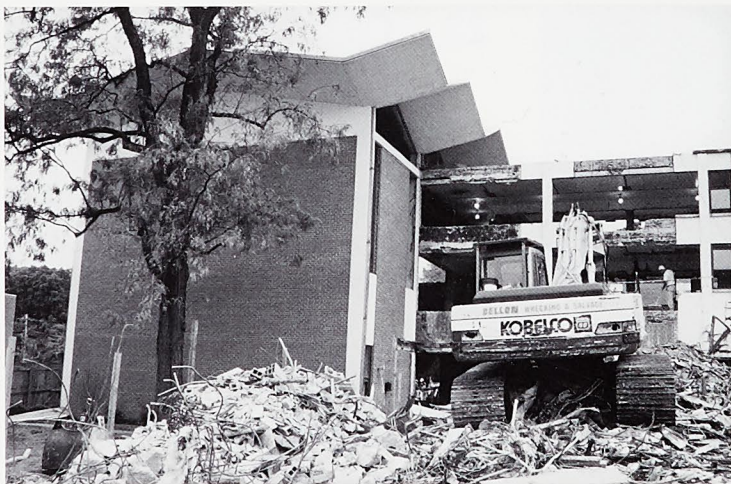
Southwest Hall gets a complete makeover.
