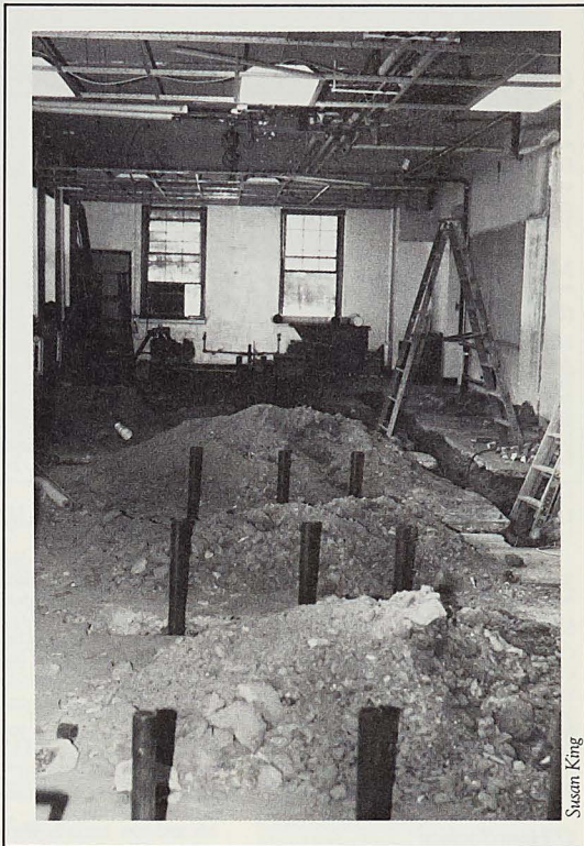
Chemistry Lab During Construction
